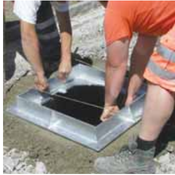
The top frame included is put on the pre-fitted concrete standard tube.
