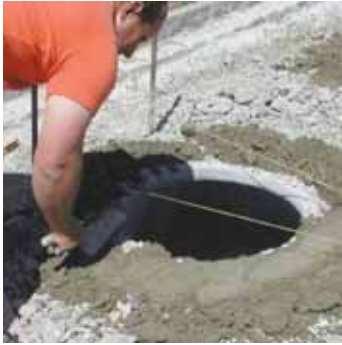
The top frame included is put on the pre-fitted concrete standard tube.
