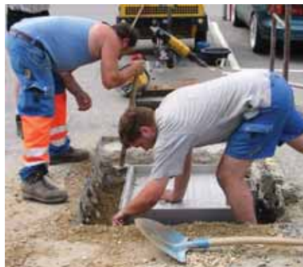
Filling around and concrete in the base socket.
