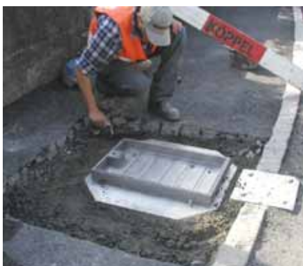
Fixing of the top cover.
