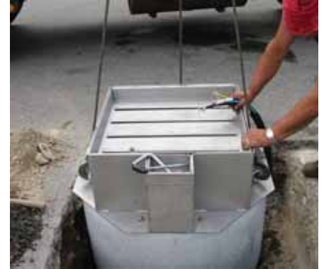
Sink the entire unit into the prepared pit using suitable equipment (crane).
