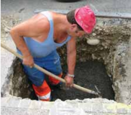
Excavation of the hole based on our specified measurements
