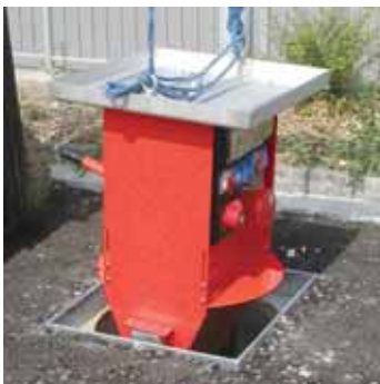
Fit the unit and screw on the guide rails.
