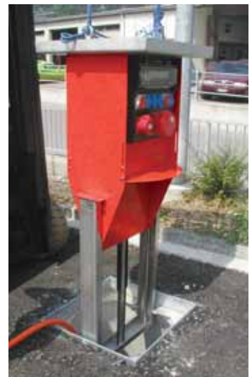
The underfloor distributor can be inserted after connecting the flexible supply line to the connection box.
