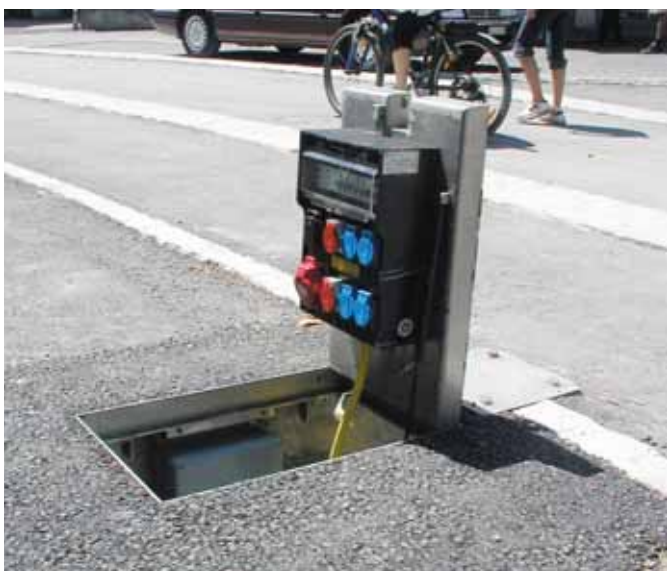
The CAMPETTO (special construction) is ready for use.
