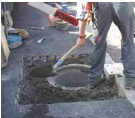
The concrete tube is installed by the customer.
