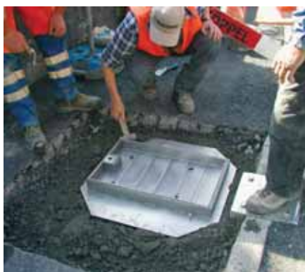
Clean underfilling, to avoid subsidence.
