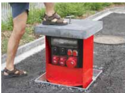
The strong gas springs prevent the underfloor distributor being retracted of their own accord.
