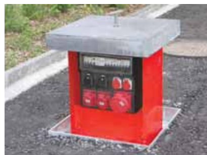
The strong gas springs prevent the underfloor distributor being retracted of their own accord.
