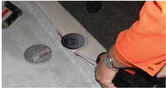
Sealing of groove with sealing compound
