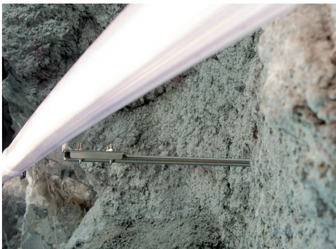
Mounting with rockbolts (details on page 8)
