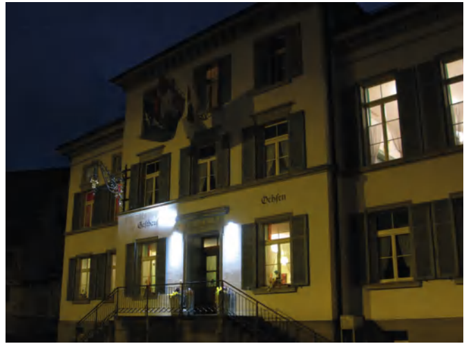
SpotLED 230V facade lighting
