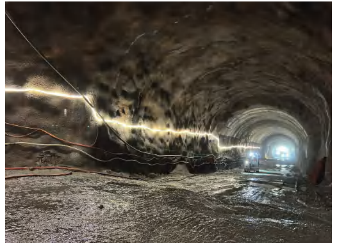
Implenia Switzerland, ARGE Gotthard
