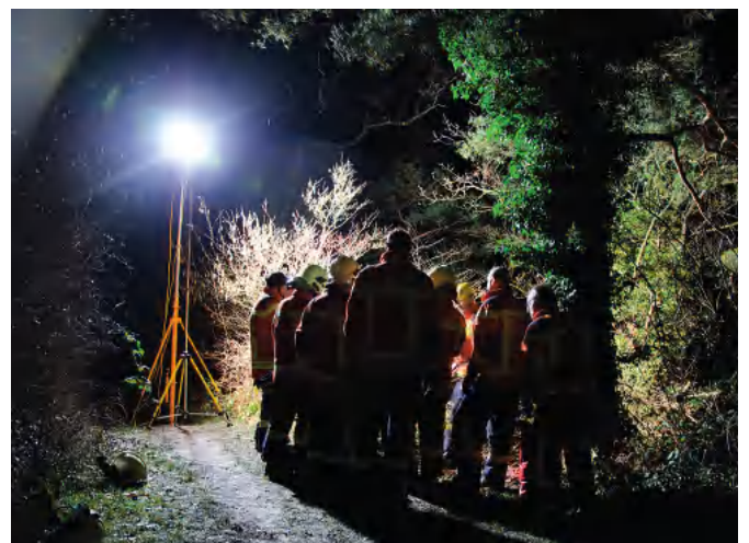
Illumination AlphaLUX during firefighter
